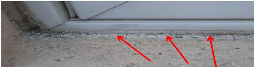
*Cracked PU(Polyurethane) Sealant
