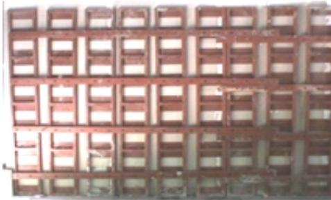
**Step 4 - Install Metal Form (Temporary Wall)**
