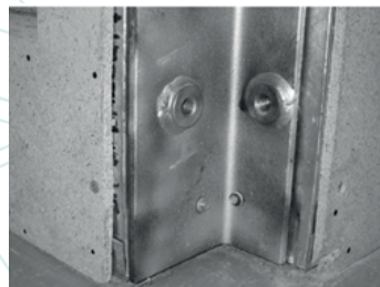
Figure 3.8: Corner angle with welded nut to connect the tie plate
