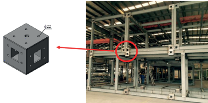
Figure 3.12: Steel bracket connection welded to corner column
